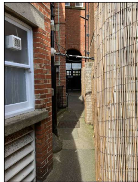
Current pedestrian access route. Obstructed from the front elevation by a permanently closed gate.
